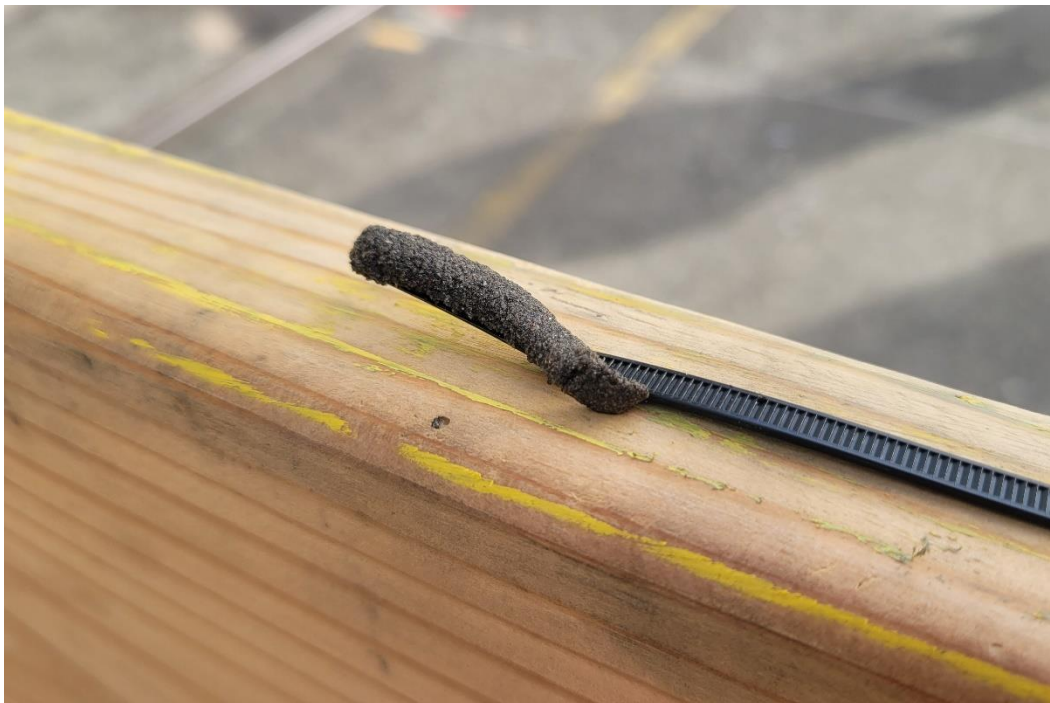
Photo 3-3 Sample of Grit Retrieved from Interior of Traversing Beam
