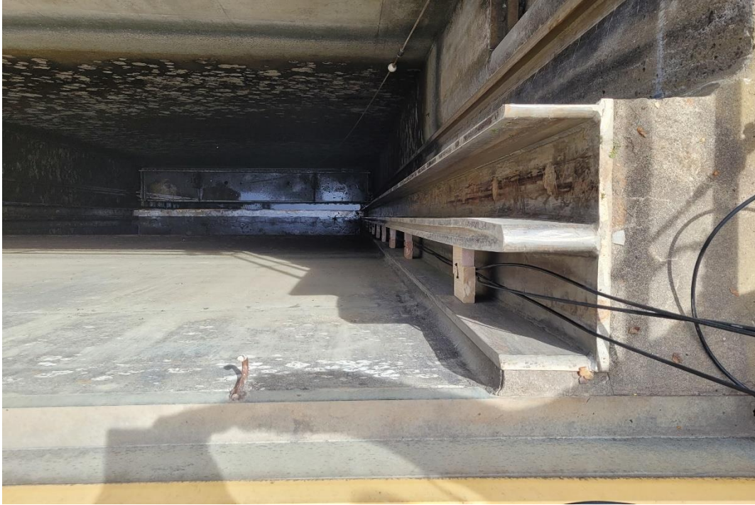
Photo 2-6 Wedges and Pressure Sensor Cable Routing in VBS Slot
