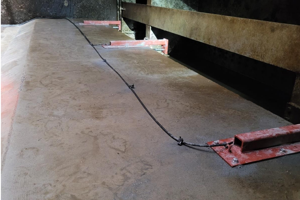
Photo 2-4 Pressure Sensors Installed in Unit 15A
