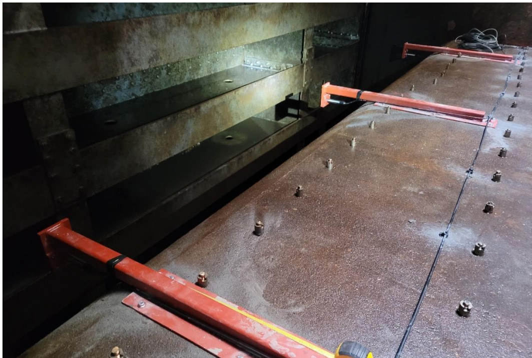
Photo 2-3 Pressure Sensors Installed in Unit 14A
