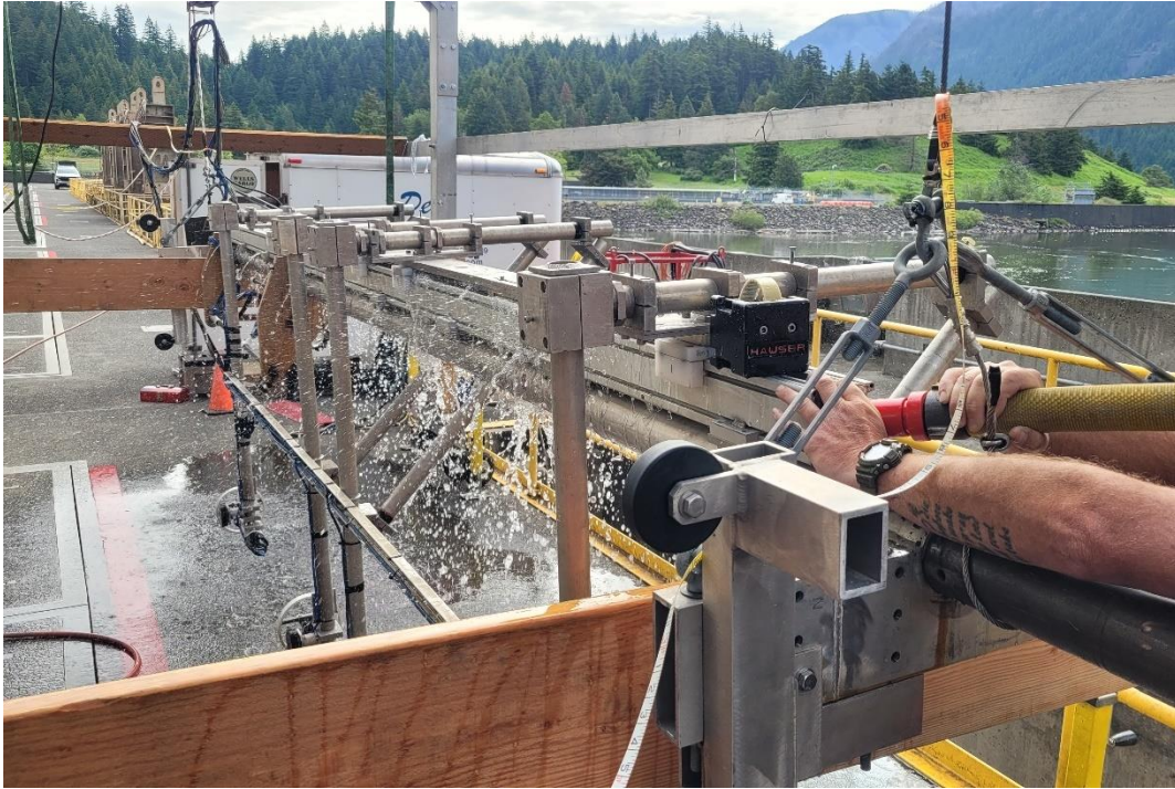
Photo 3-4 Flushing of Grit from Traversing Beam (End View)
