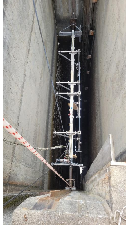
Photo 2-12 Traversing Beam Deployed in Gatewell
