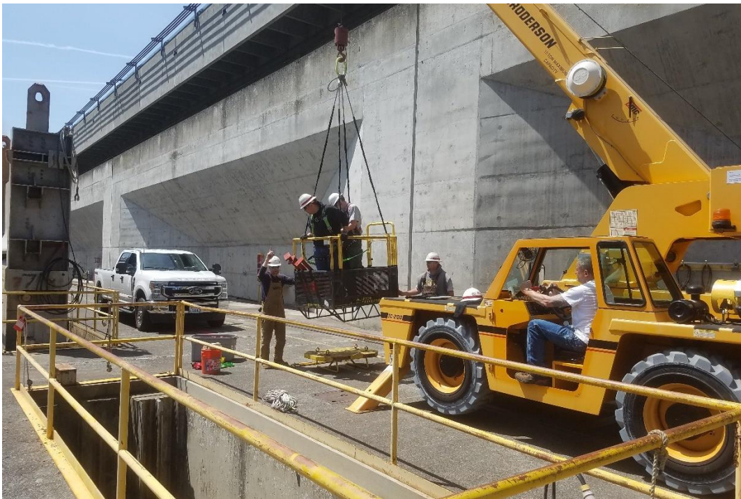
Photo 2-7 Crane and Man-Basket used for Pressure Sensor Installation
