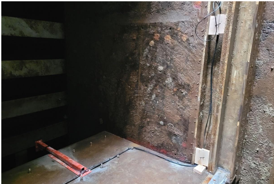
Photo 2-5 Pressure Sensor Cable Routing to Downstream VBS Slot – Unit 14A
